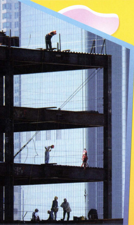
A strong steel frame will hold up this skyscraper.
